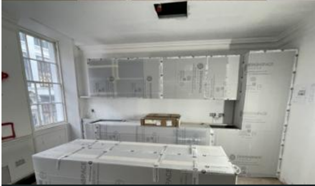
Newly installed kitchens
