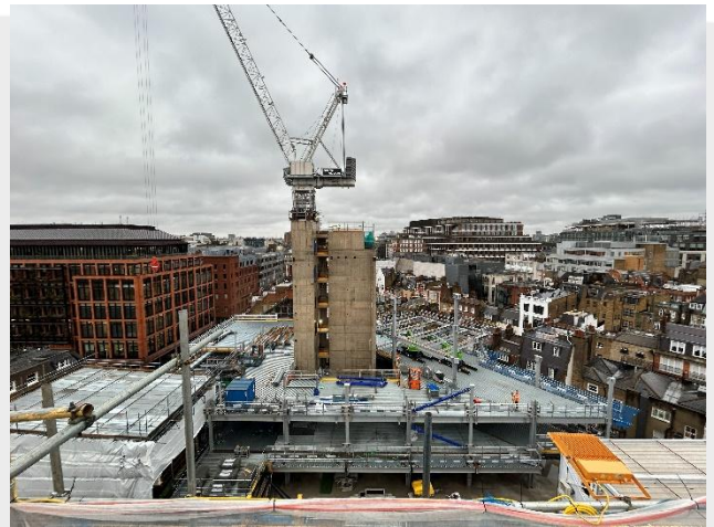
North Building Progress
