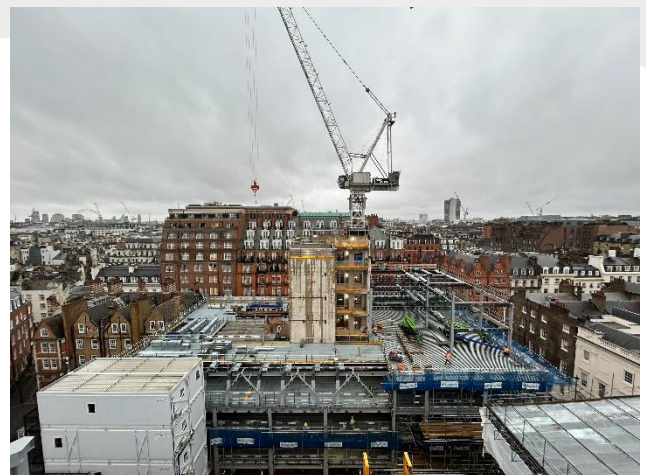
South Building Progress
