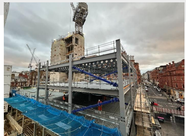
South Block Steel Frame and Metal Deck Progress
