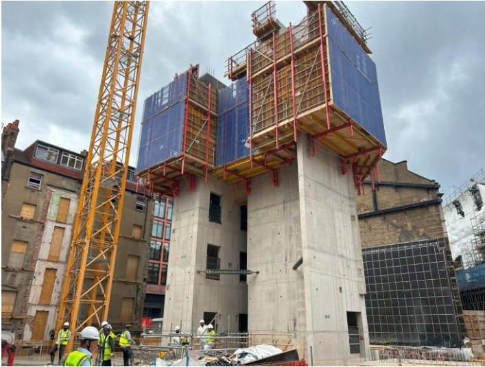
North concrete core structure
