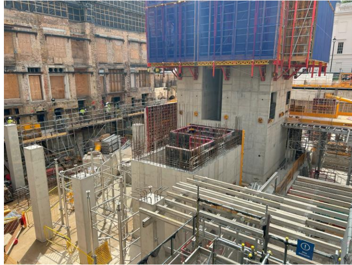
Small core poured to ground floor level
