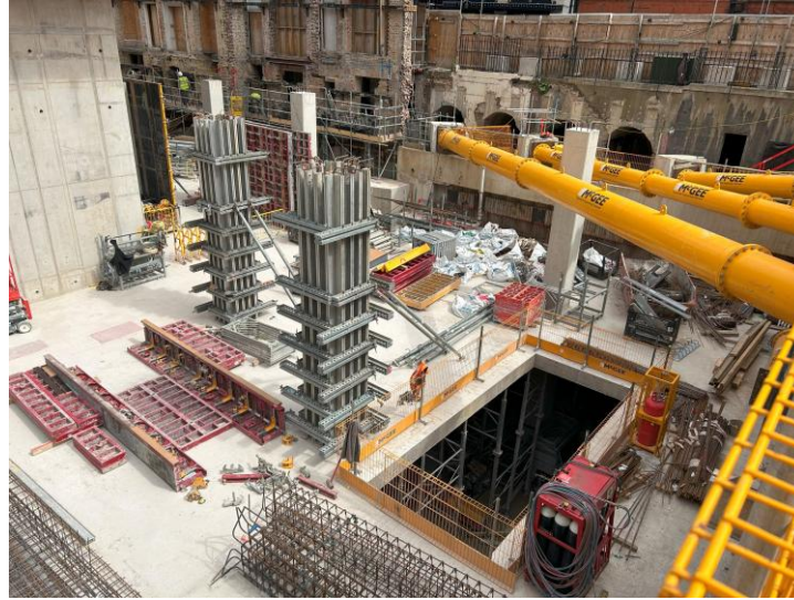
Pouring of reinforced concrete columns
