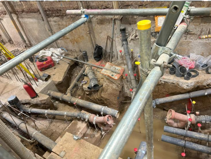
Basement drainage install in the RHP
