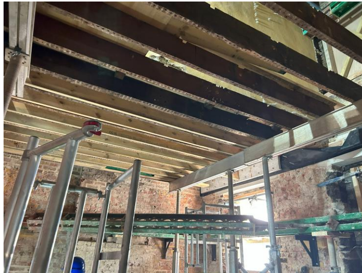
Floor joist strengthening in the RHP
