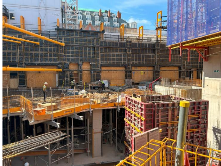
Decking and fixing of the first GF slab pour
