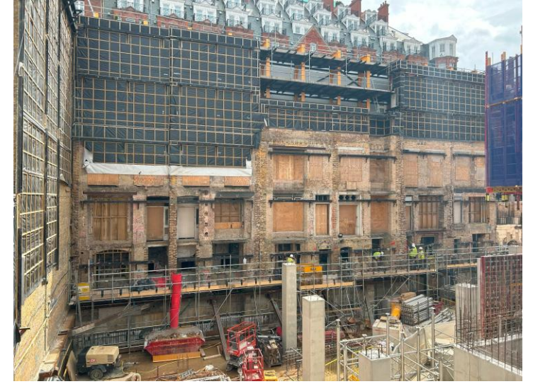
Brook street façade restoration works
