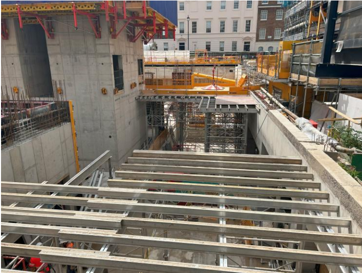
Ground floor falsework erection
