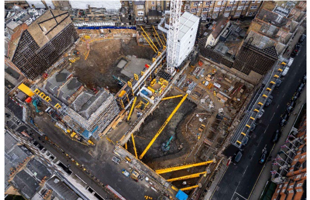
Site Overview including excavation progress
