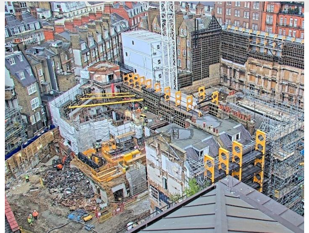
Site Overview including demolition progress
