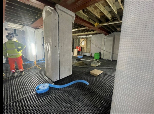
Waterproofing Basement of 15 and 16 progressing
