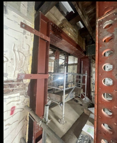
New structural steel picture frame installed in 18 and 19
