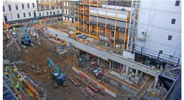
Davies Mews ground floor completion
