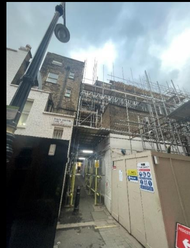
Scaffolding progress down South Molton Lane
