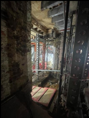
Wall knock through between 18 and 19 SMS
